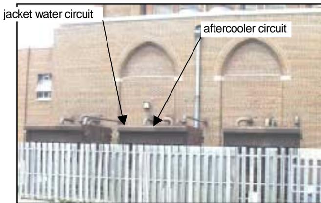
**Figure 7: Engine Radiators (Amercool Mfg., Inc.)
