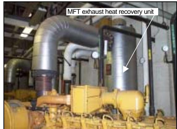
**Figure 6: Beaird Industries MFT exhaust heat recovery unit (one/engine/gen set). Each one produces 1000-1200 lb/hr of 100-110 psig steam**
