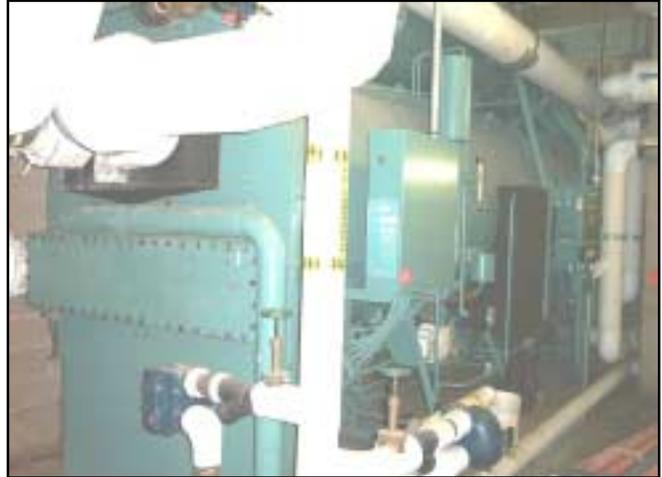
**Figure 10: One of Four Existing York 520-Ton Single-Stage Steam-Fired Absorption Chillers**
