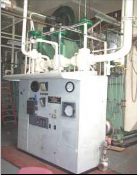
**Figure 9: One of Three Existing Steam Boilers (Babcock & Wilcox 50,000 lb/hr design output)**
