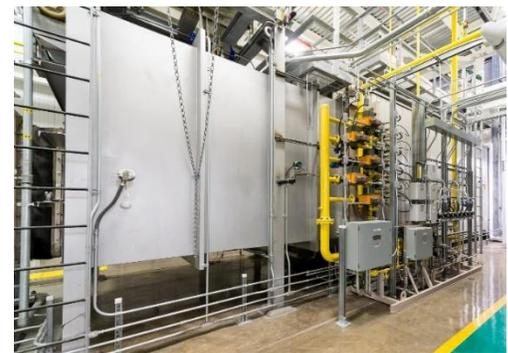
**HRSG with Side Mounted Duct Burners**
